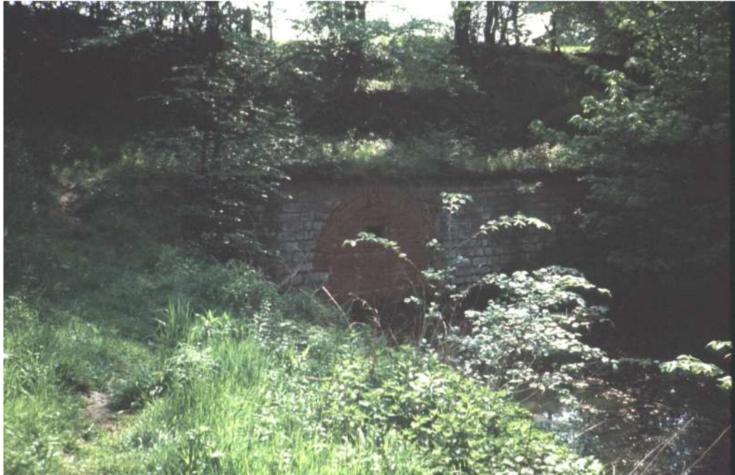
Figure 8.12.1 Norwood Tunnel Western Portal.
