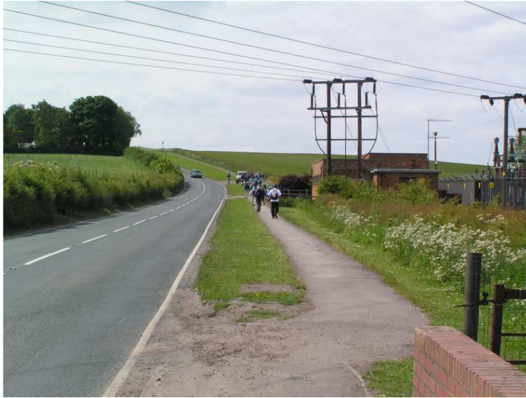
View along Hard Lane Looking south towards Harthill.
