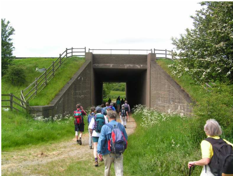
Poplar Farm Underpass under the M1 Motorway. Looking west.
