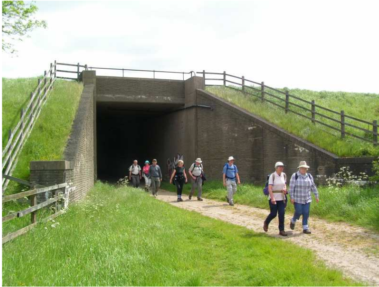
Poplar Farm Underpass under the M1 Motorway. Looking east.
