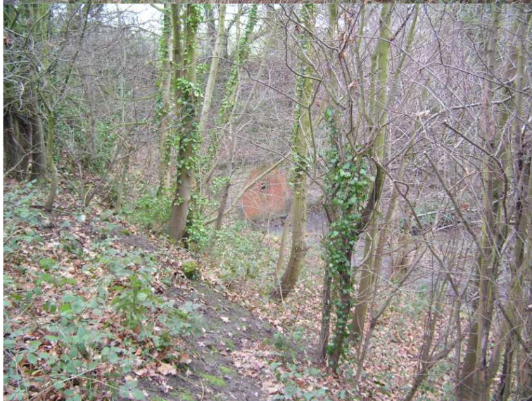
Norwood Tunnel West Portal seen through woodland, looking east.
