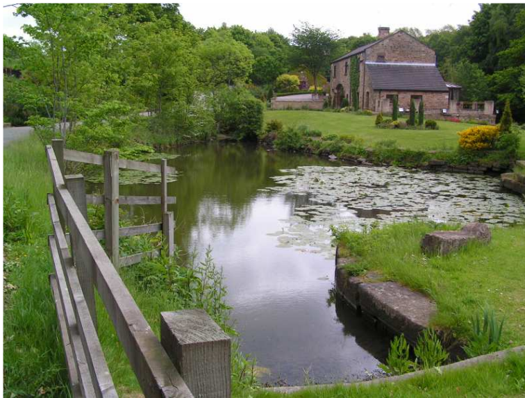
The former Norwood Sawmill (now a private house) looking east.
