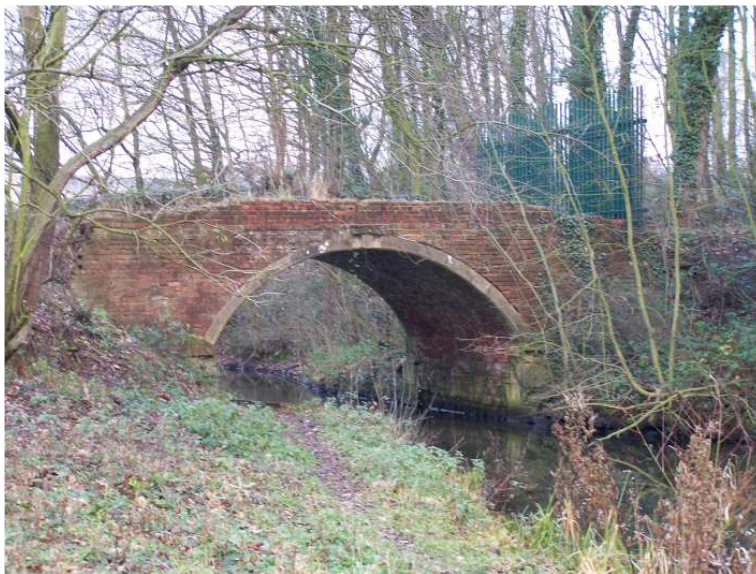
Norwood Bridge (No.30) looking east.
