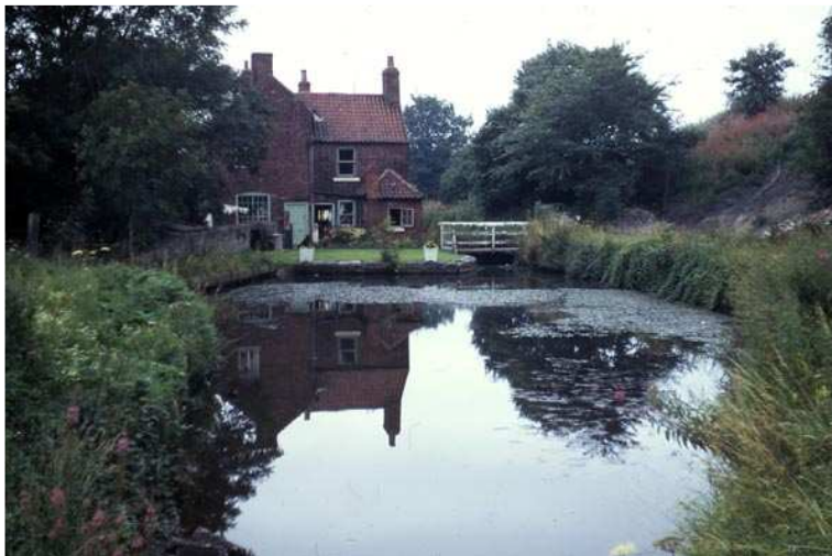
Norwood Lock Keepers House in 1972, looking west.
