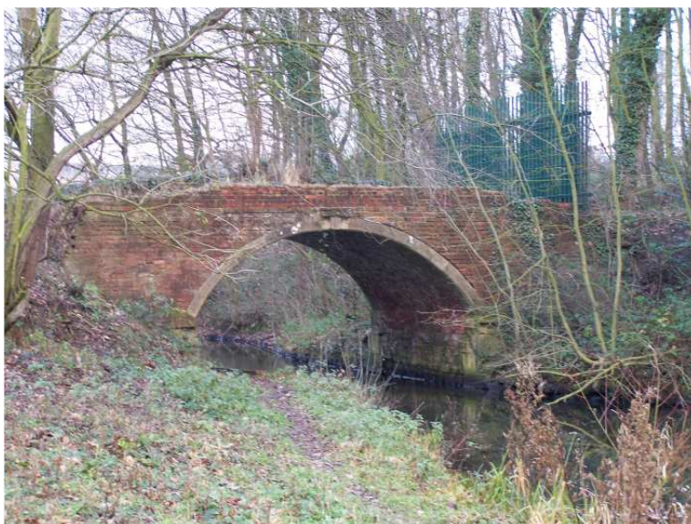
Norwood Bridge looking east.
