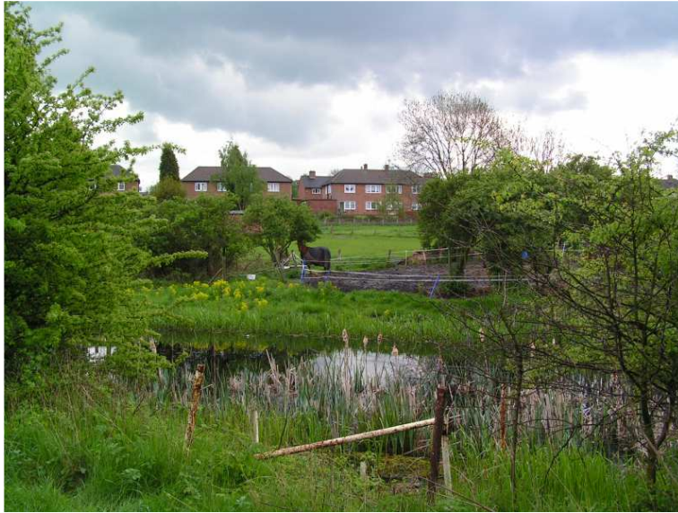
View of canal channel at Norwood Bends looking south.
