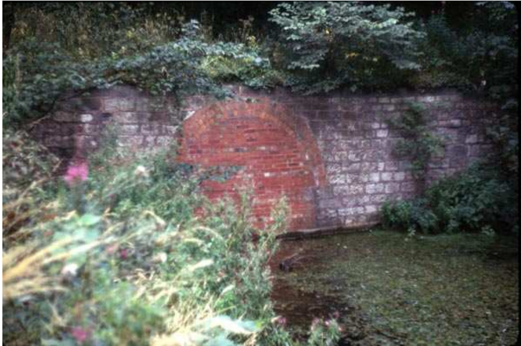
Figure 14.2 Norwood Tunnel Eastern Portal
