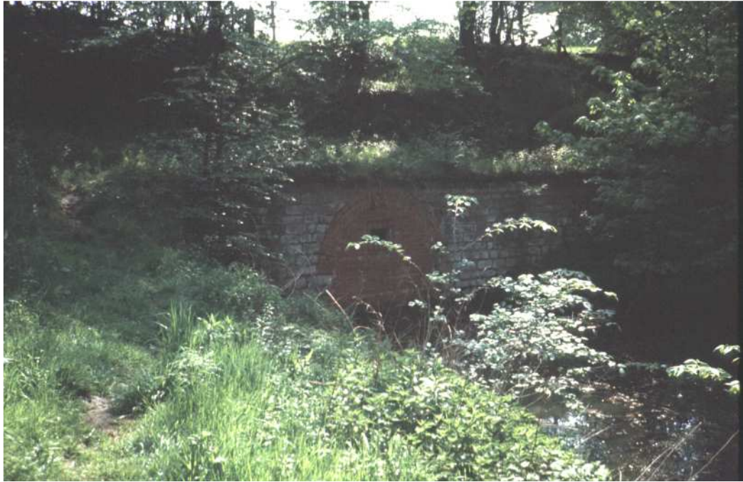
Figure 14.1 Norwood Tunnel Western Portal
